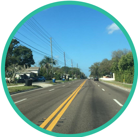
Lack of Mid-Block Crossings
