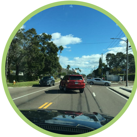
Lack of Left-Turn Lanes
