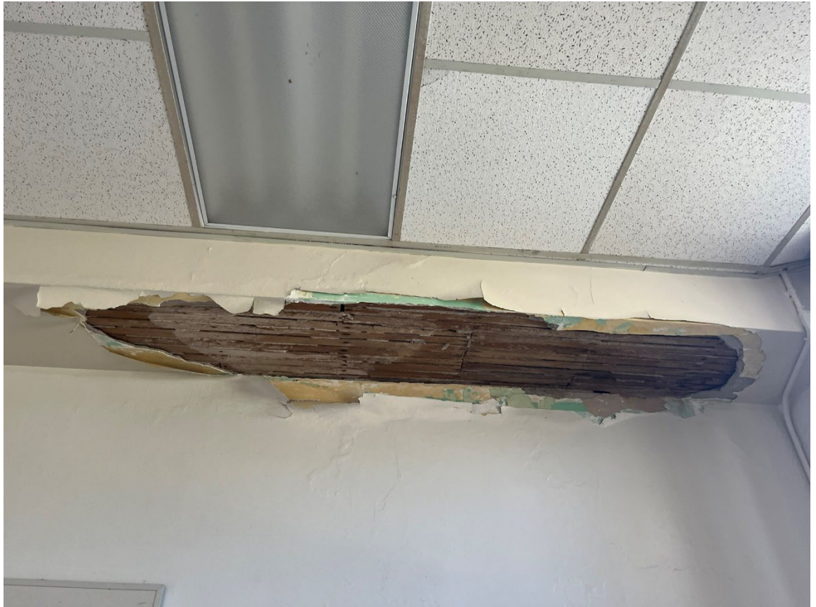
Figure 6 – Building 1 water damage
