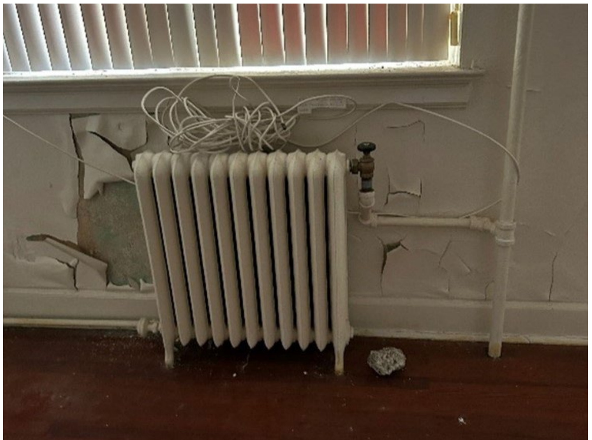
Figure 83 – Existing cast iron steam radiator
