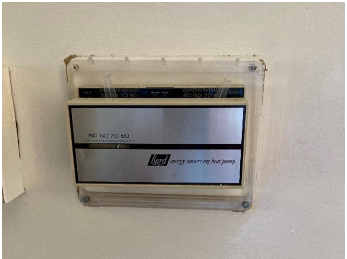
Figure 85 – Existing thermostat, 24/7 programmable
