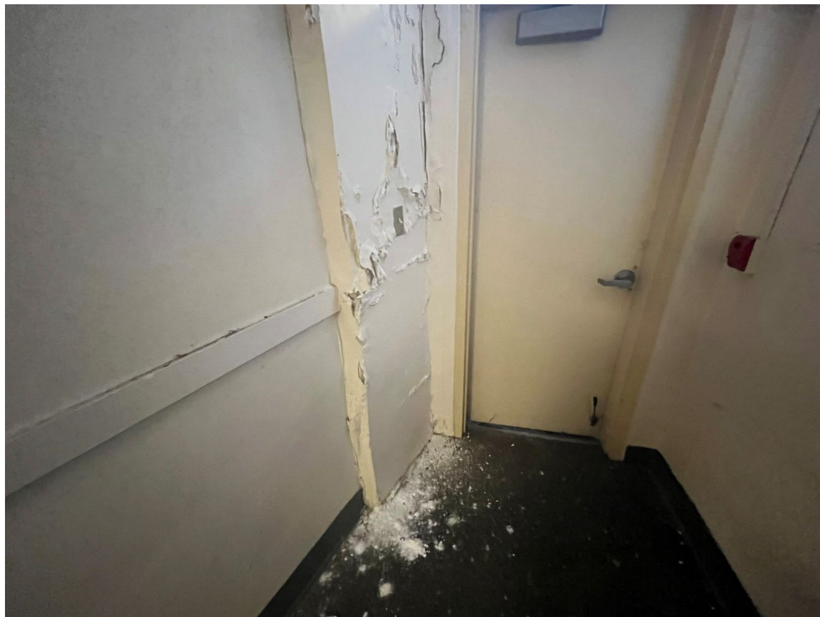
Figure 58 – Building 3 moisture damage
