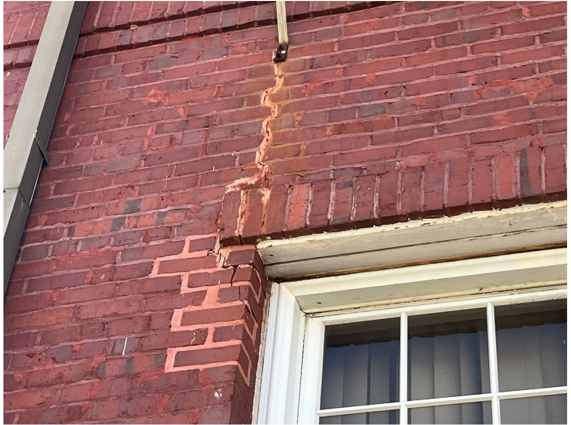
Figure 11 – Building 1 step cracking
