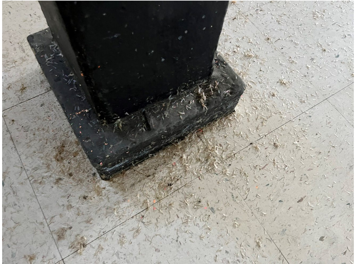
Figure 63 – Building 4 termite activity
