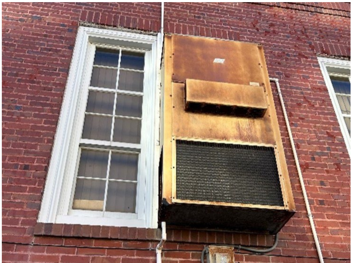
Figure 81 – Existing packaged direct expansion wall-hung air handling unit
