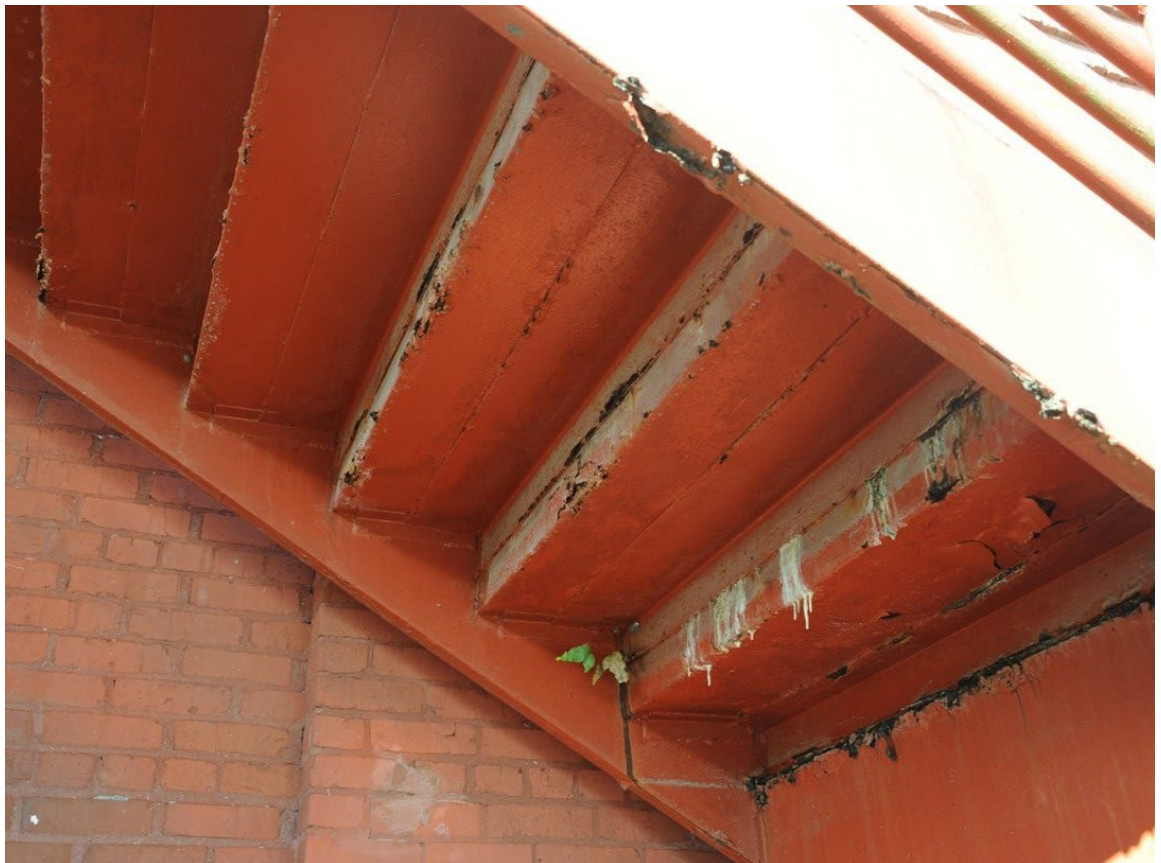
Figure 70 – View of corroded metal pan stair
