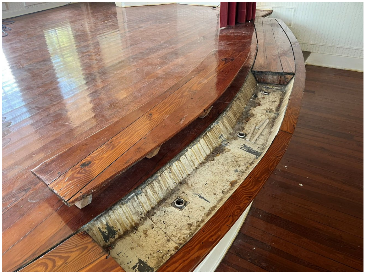
Figure 29 – Building 1 stage light trough
