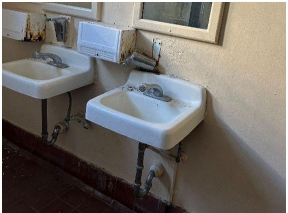
Figure 76 – Existing Lavatories with self-closing faucets
