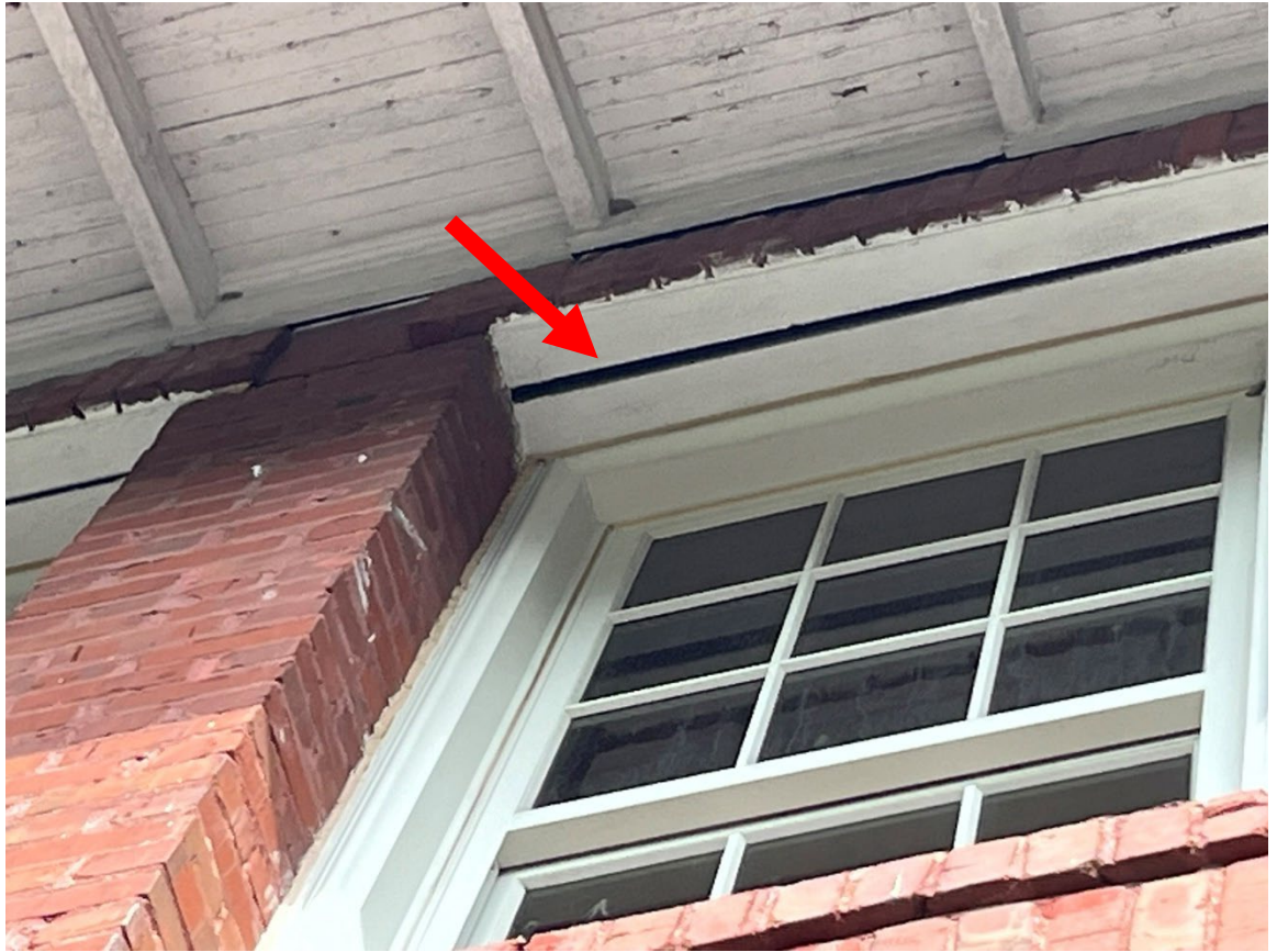
Figure 17 – Building 1 window lintels
