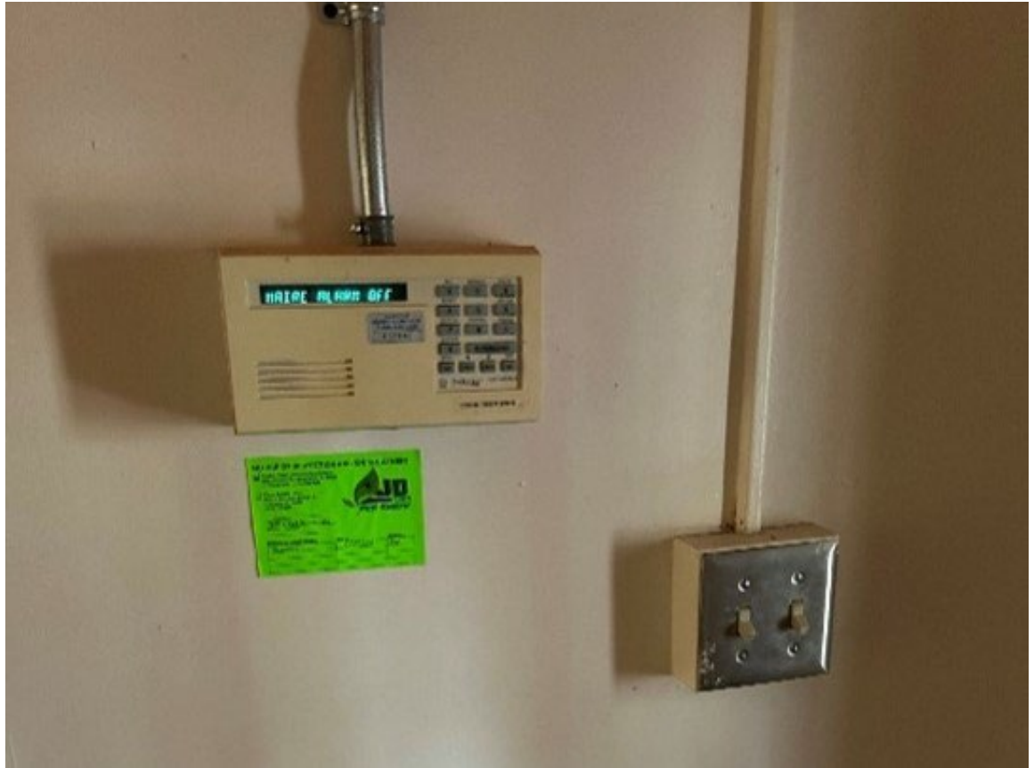
Figure 98 – Security system keypad
