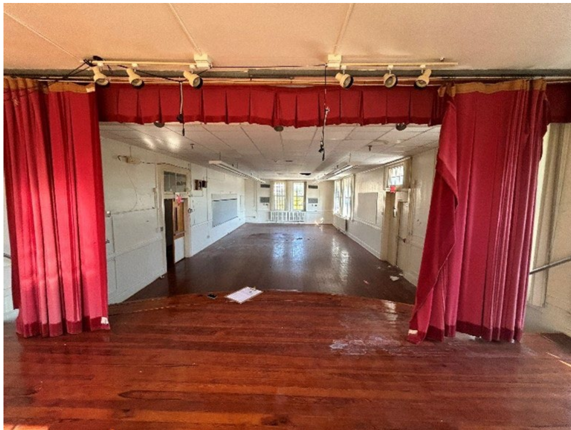
Figure 91 – Stage Spotlights and Fluorescent Pendant Lighting
