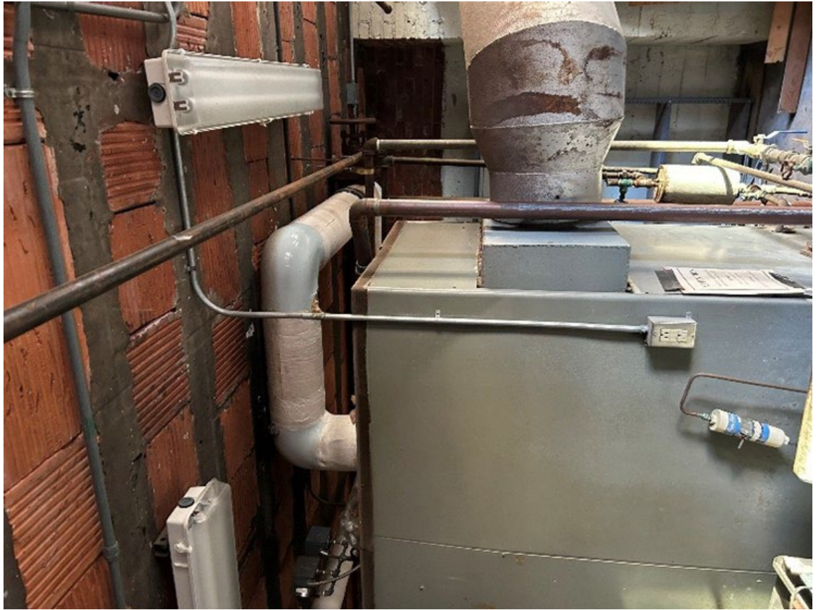
Figure 82 – Existing gas-fired steam boiler
