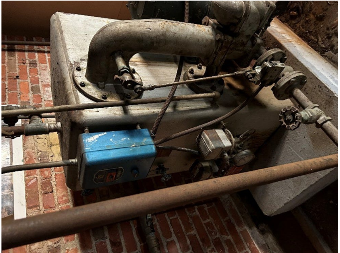
Figure 80 – Existing condensate return pump
