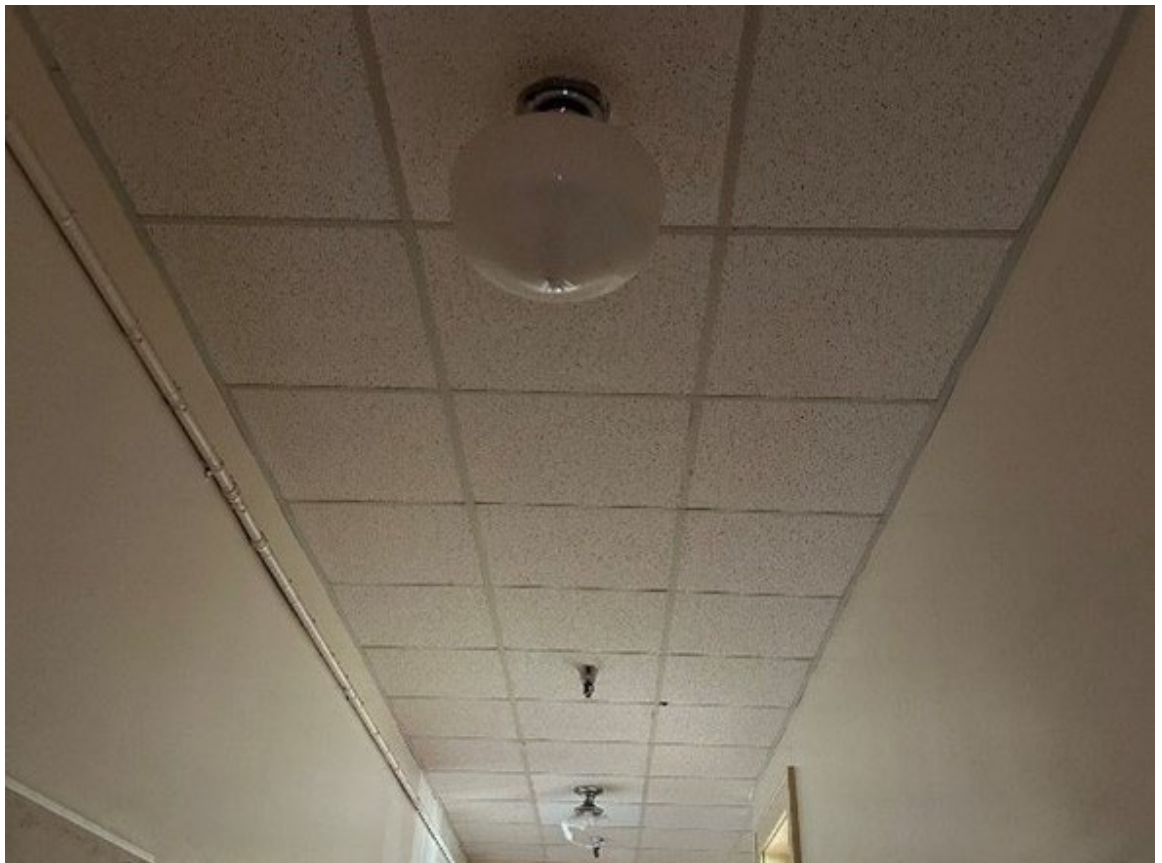
Figure 90 – Incandescent Schoolhouse Luminaires in Corridor
