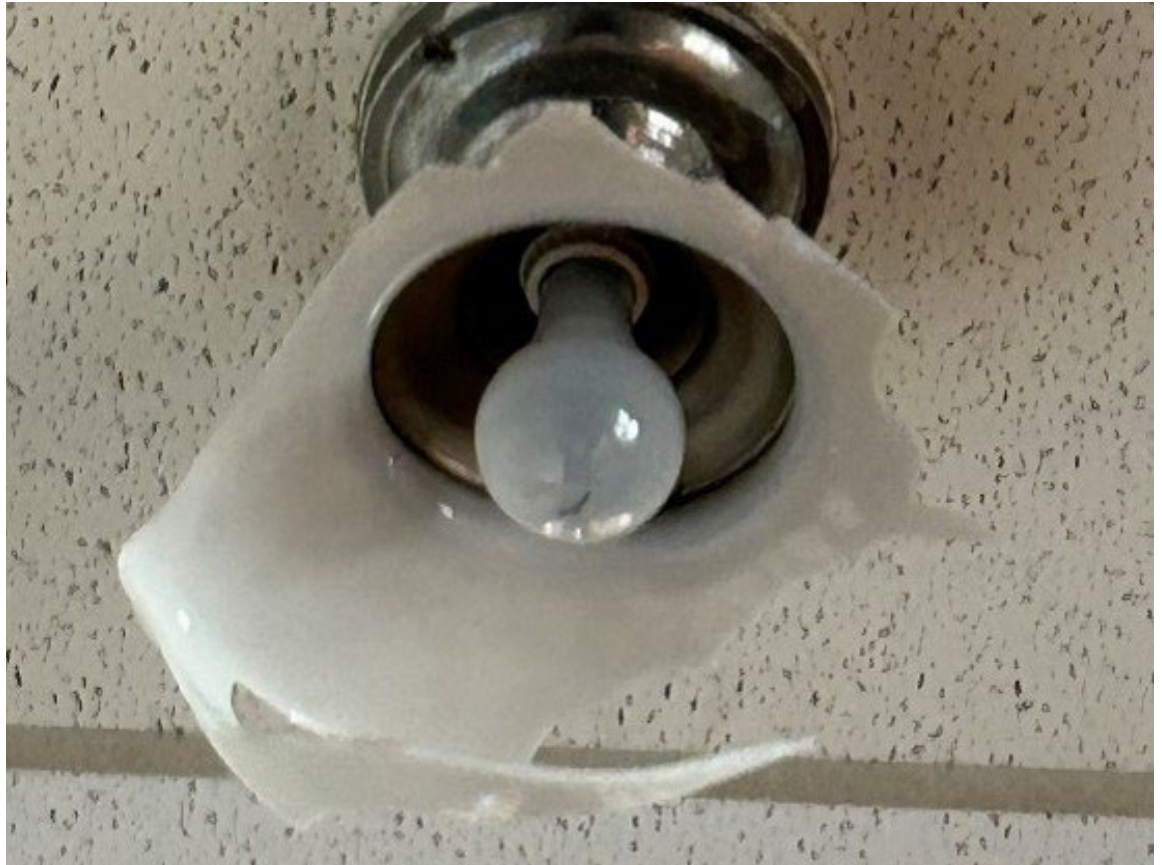
Figure 89 – Incandescent Schoolhouse Luminaire (broken)
