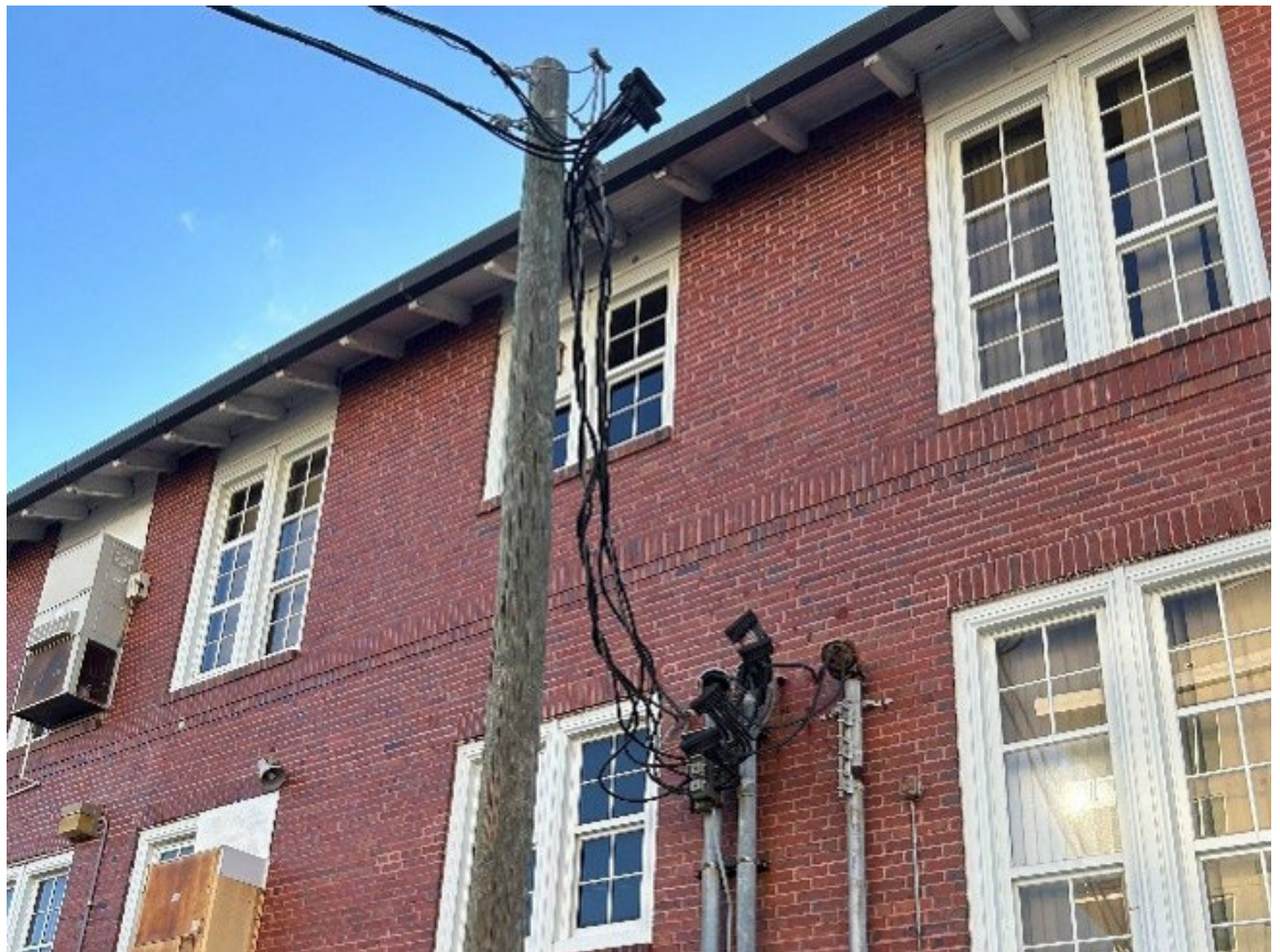
Figure 87 – Electrical Service Drop on West Wall of Building 1
