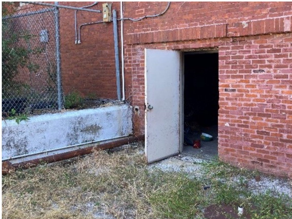
Figure 79 – Existing exposed fire protection pipe
