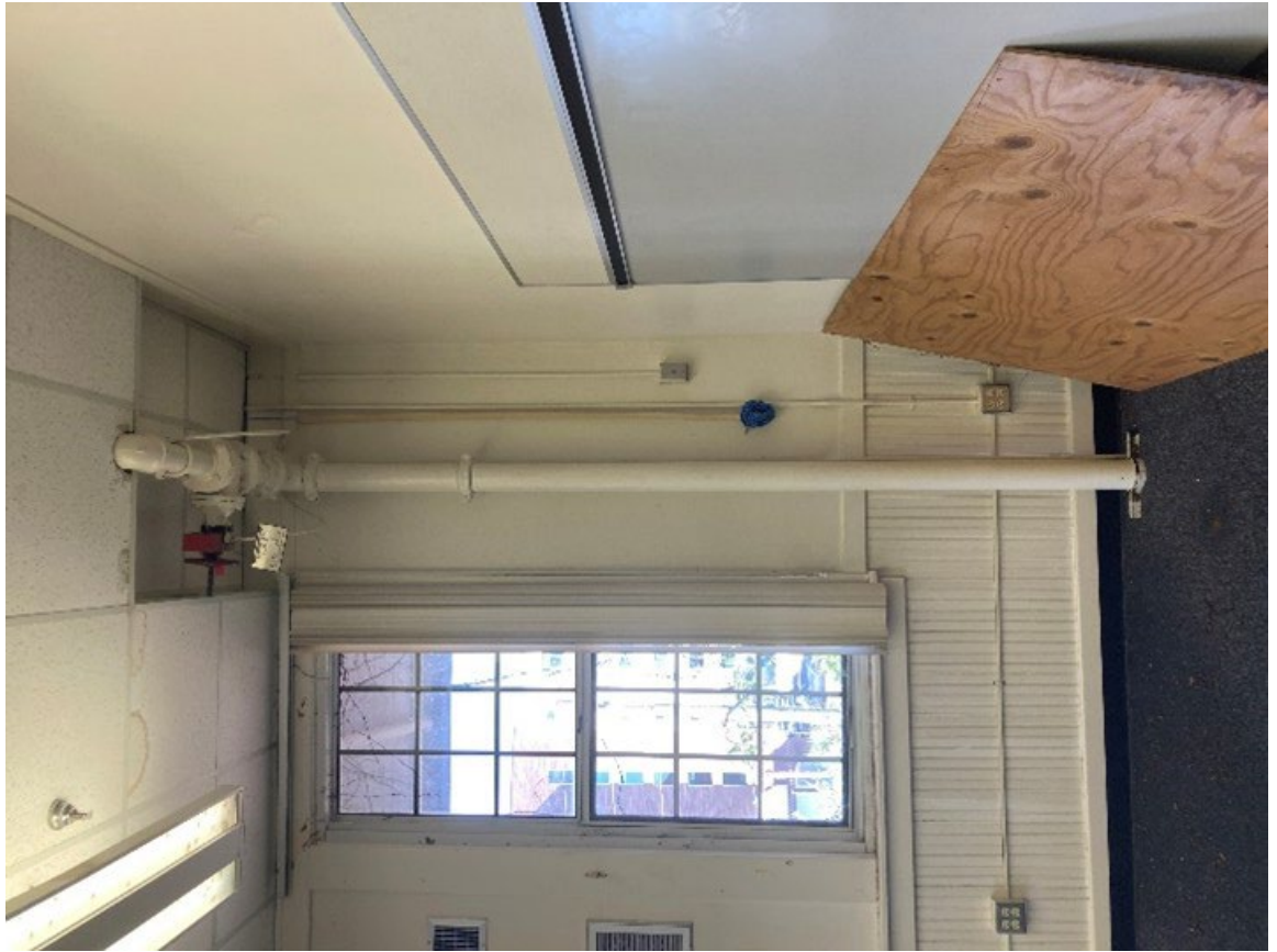
Figure 77 – Sprinkler riser in Building 1
