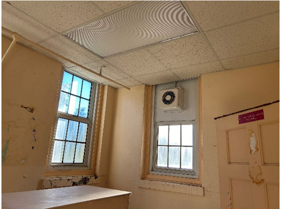
Figure 84 – Existing bathroom exhaust fan
