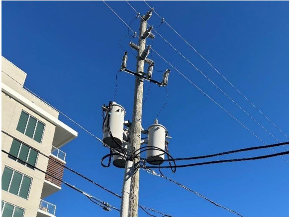
Figure 86 – Duke Energy pole-mounted transformers
