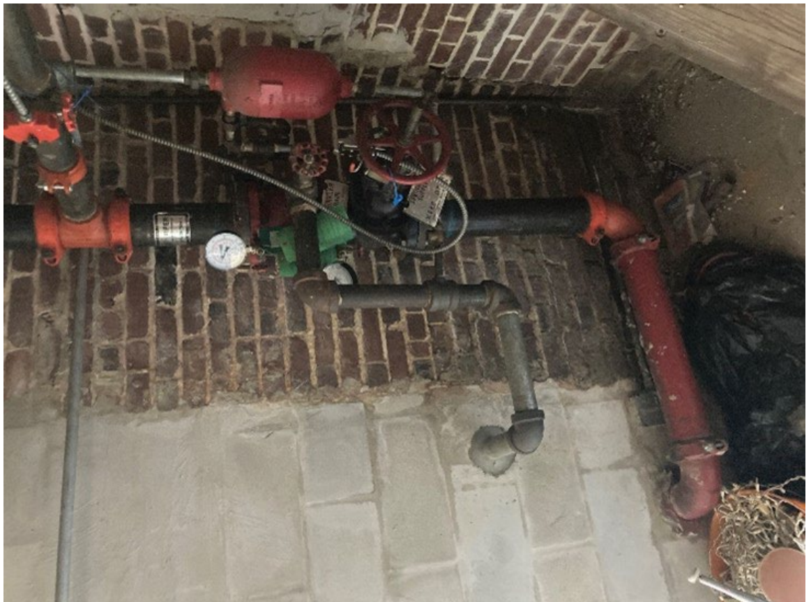
Figure 78 – Main sprinkler riser in Building 2 basement
