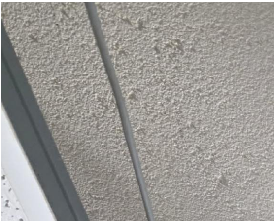
Photo #3 AHU C, Off White Acoustical Texture Ceiling Texture
