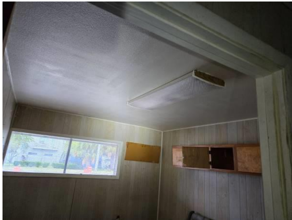
Photo #1 AHU C, Off White Acoustical Texture Ceiling Texture
