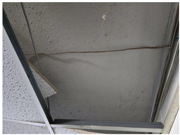
Photo #2 AHU C, Off White Acoustical Texture Ceiling Texture
