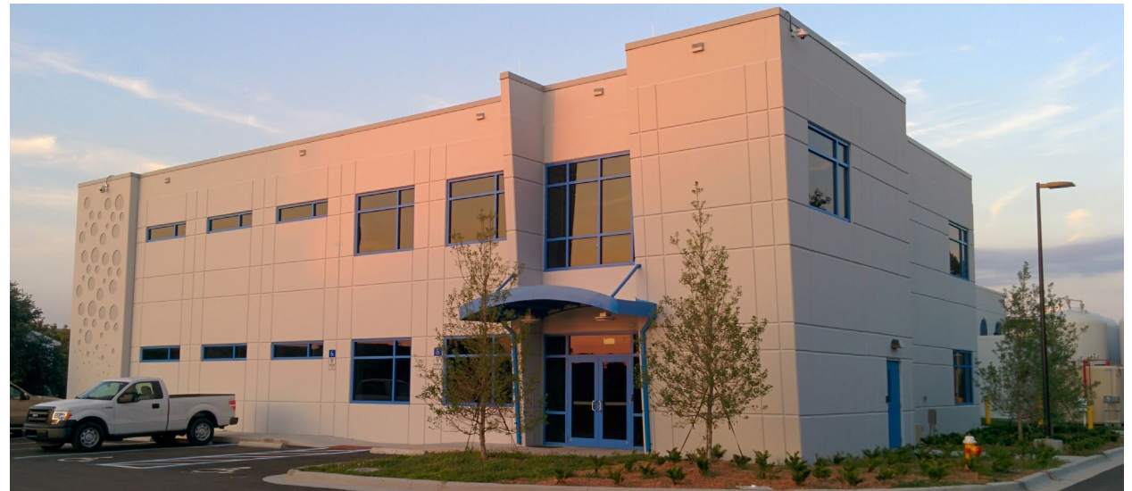
Reverse Osmosis Plant #2
