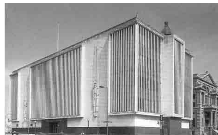
Before - Tarrant County Court-house, Ft Worth, TX
