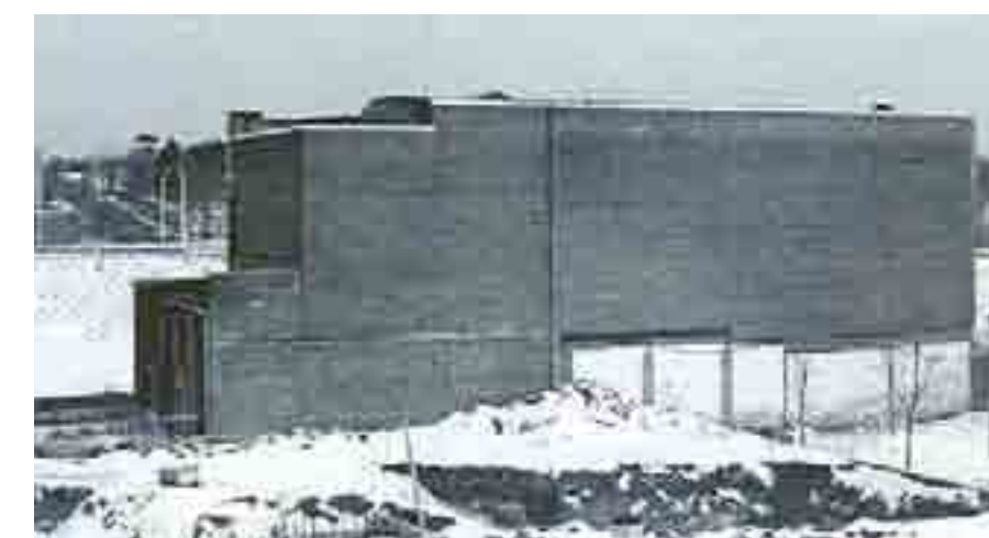
Before - P.S.E. & G. Electric Sub-station, New Brunswick, NJ
