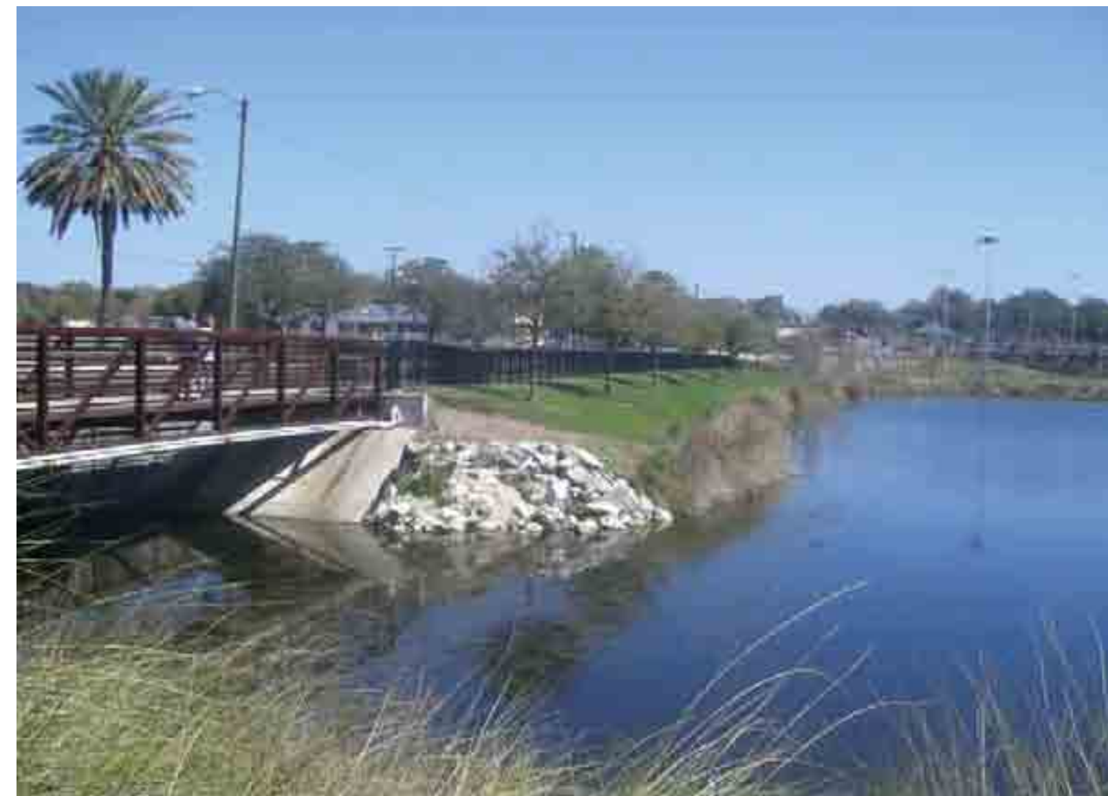
Glenn Oaks Bridge
