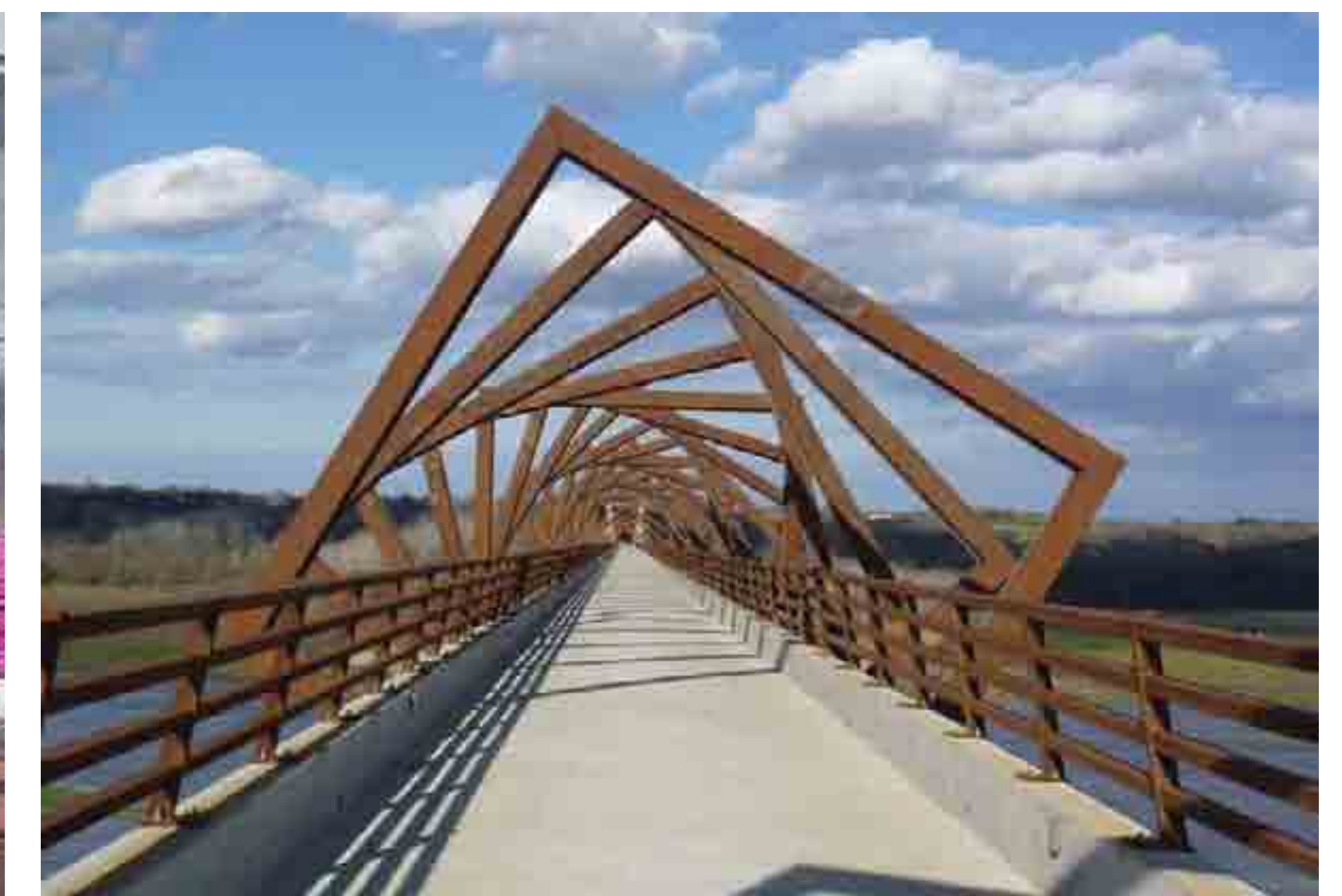
Metal Frame & Concrete Bridge
