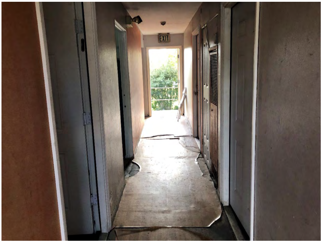
Photograph 19 – General interior view of the 2-story building, second floor residence
