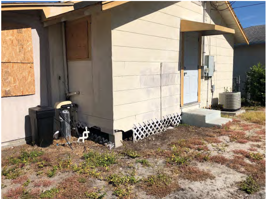
Photograph 6 – Rear door of the residence
