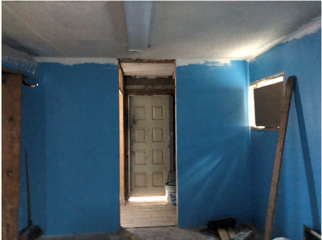
Photograph 14 - General interior view of the 2-story building, first floor commercial
