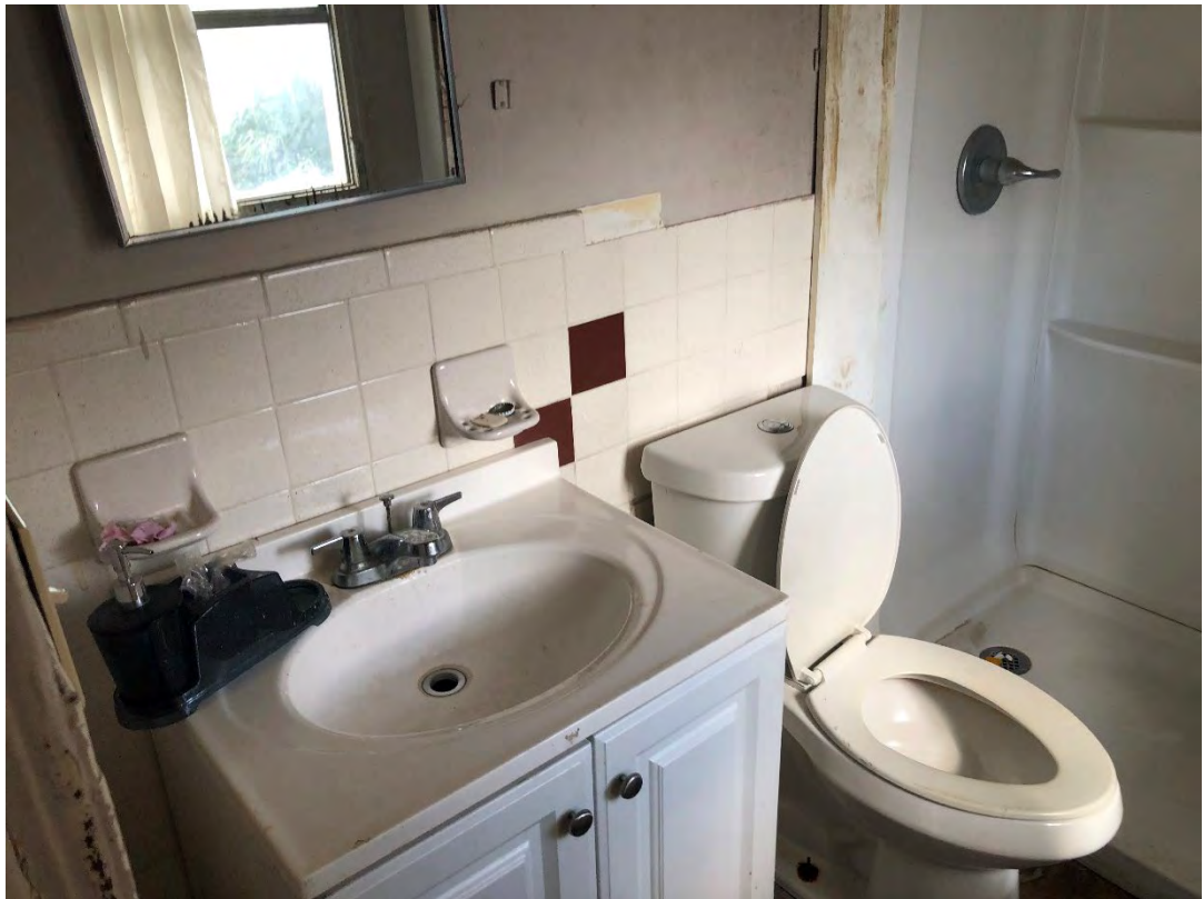
Photograph 16 – General interior view of the 2-story building, second floor residence
