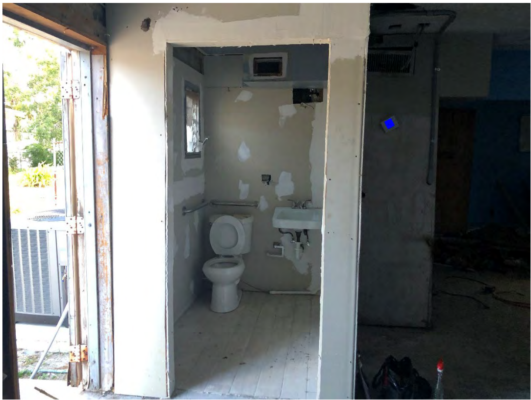
Photograph 13 - General interior view of the 2-story building, first floor commercial
