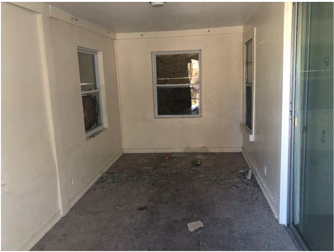
Photograph 7 - General interior view of the residence, porch
