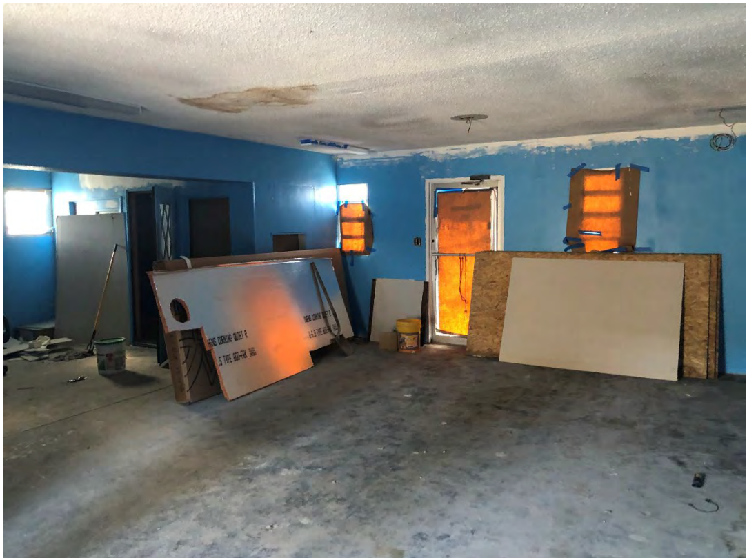
Photograph 12 – General interior view of the 2-story building, first floor commercial
