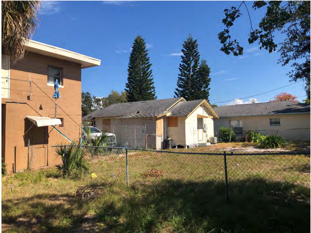
Photograph 4 – Rear of the residence facing northeast
