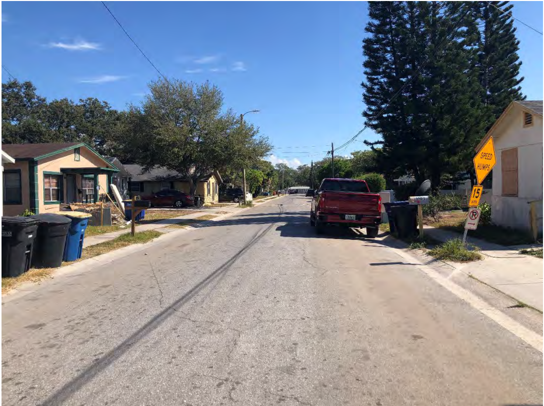
Photograph 22 - View to the east along Carlton Street
