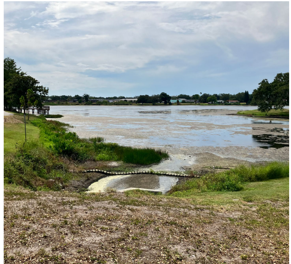
WATERGOAT stormwater system at Lake Bellevue
