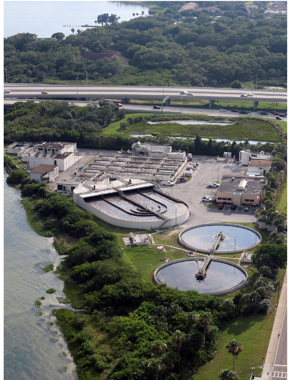
East Water Reclamation Facility
