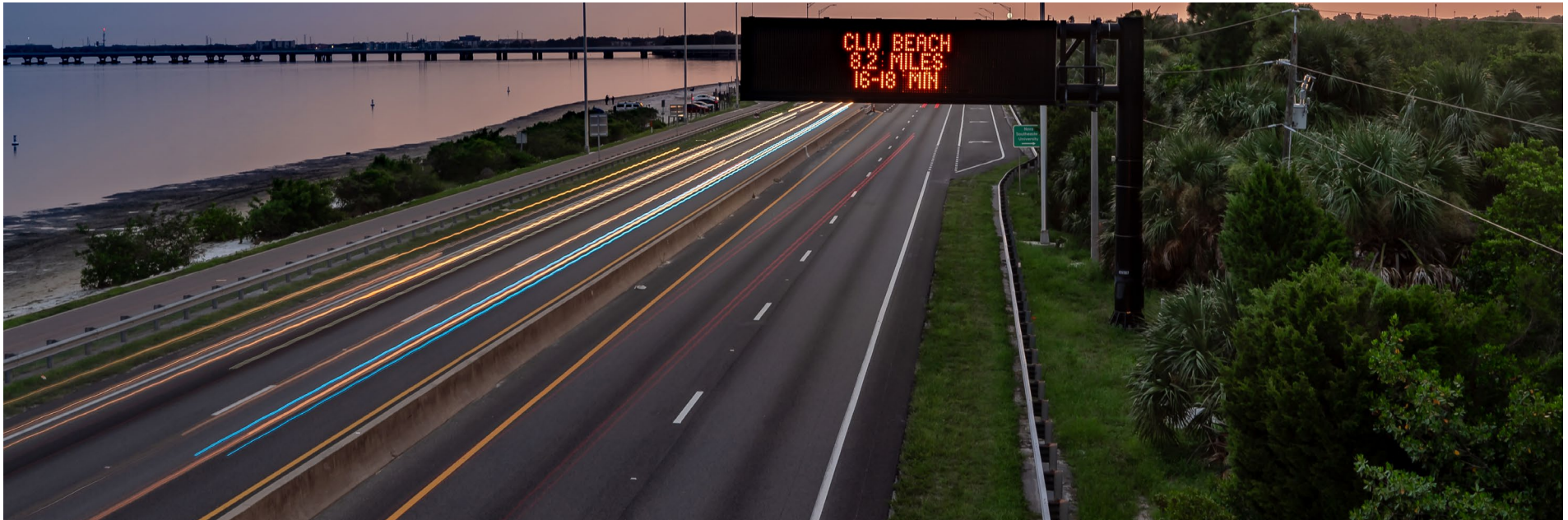
Courtney Campbell Causeway looking west. Photo credit: Pinellas County
