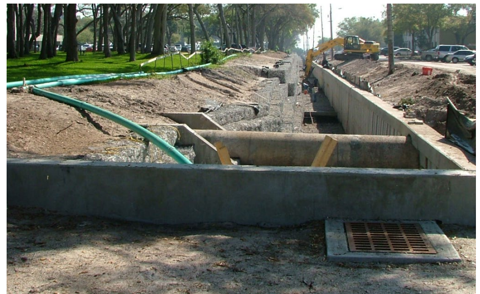
Construction of a stormwater system
