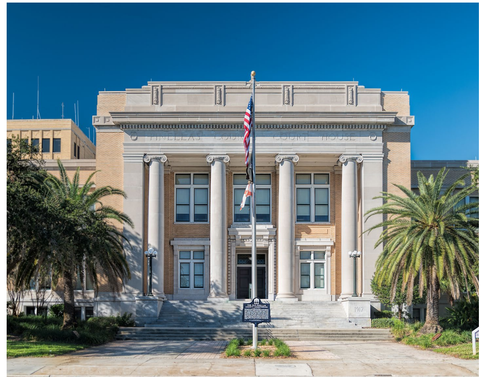
Old Pinellas County Courthouse
