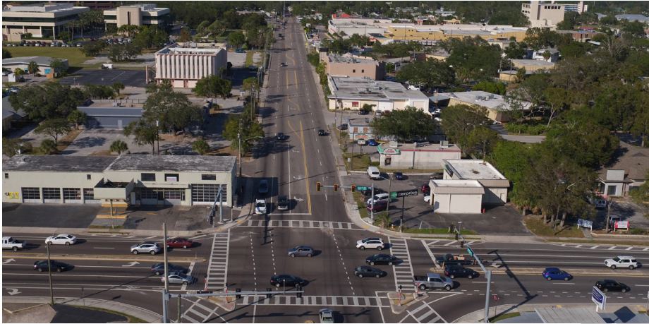
Missouri Avenue and Court Street Intersection
