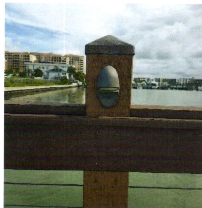
AZEK Accent LED post-mounted light fixture provided by the developer.
