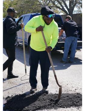
Made from bituminous limestone mined in Texas, RockAsphalt requires no heating and remains usable indefinitely, unlike traditional patches. It also comes with a three-year guarantee -- if a patch fails, the company provides a free replacement, and the warranty restarts.
