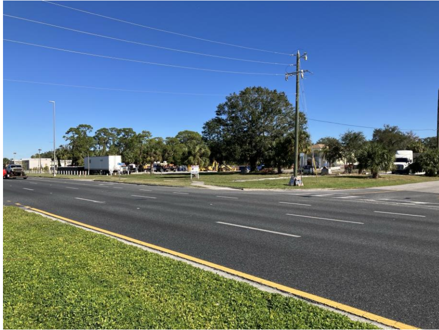
SITE VIEW LOOKING NORTHEAST FROM AVERY ROAD
