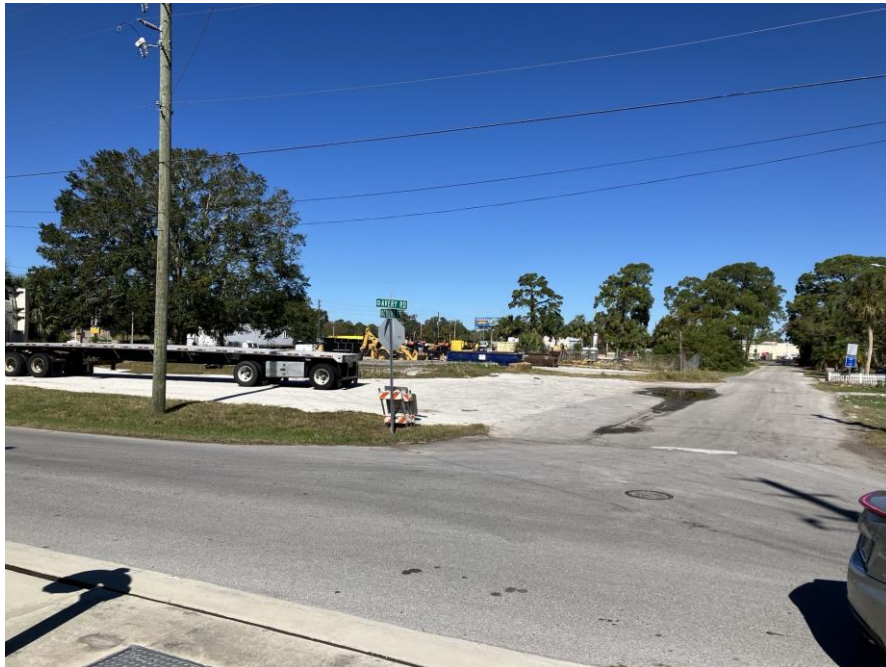
COURT STREET SCENE LOOKING NORTH FROM AVERY ROAD
