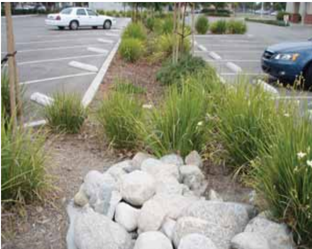
Parking lot runoff is captured in this bioswale.
