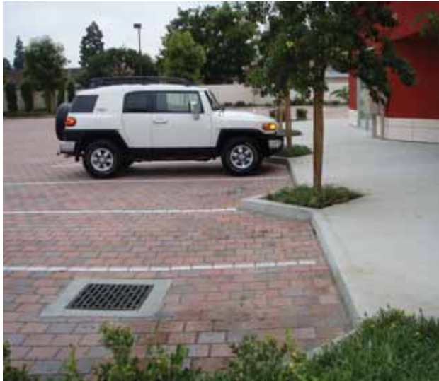
Pervious pavers with pea gravel over an infiltration area.
