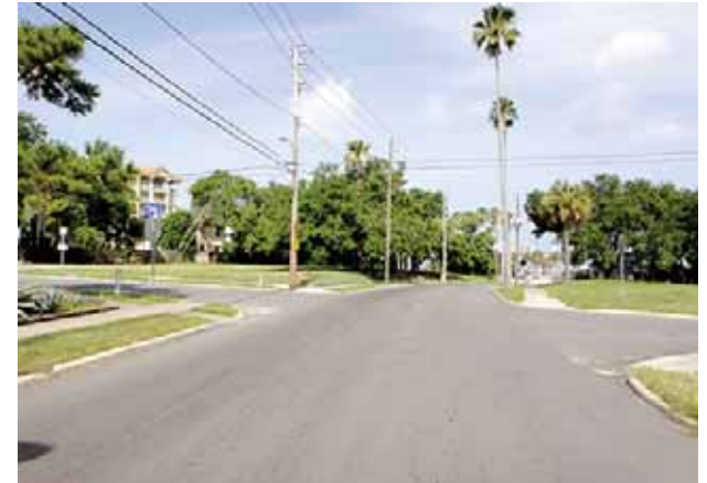
View from Osceola Avenue at Seminole Street Looking West
